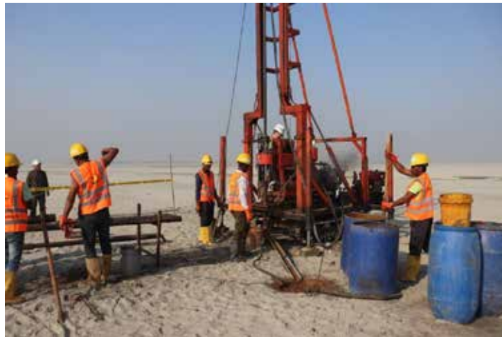
Figure 18: The drill rig in operation on exposed sandbar
