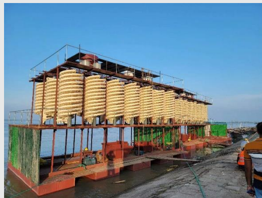
Floating wet plant
