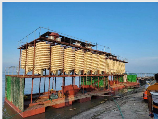
Floating wet plant
